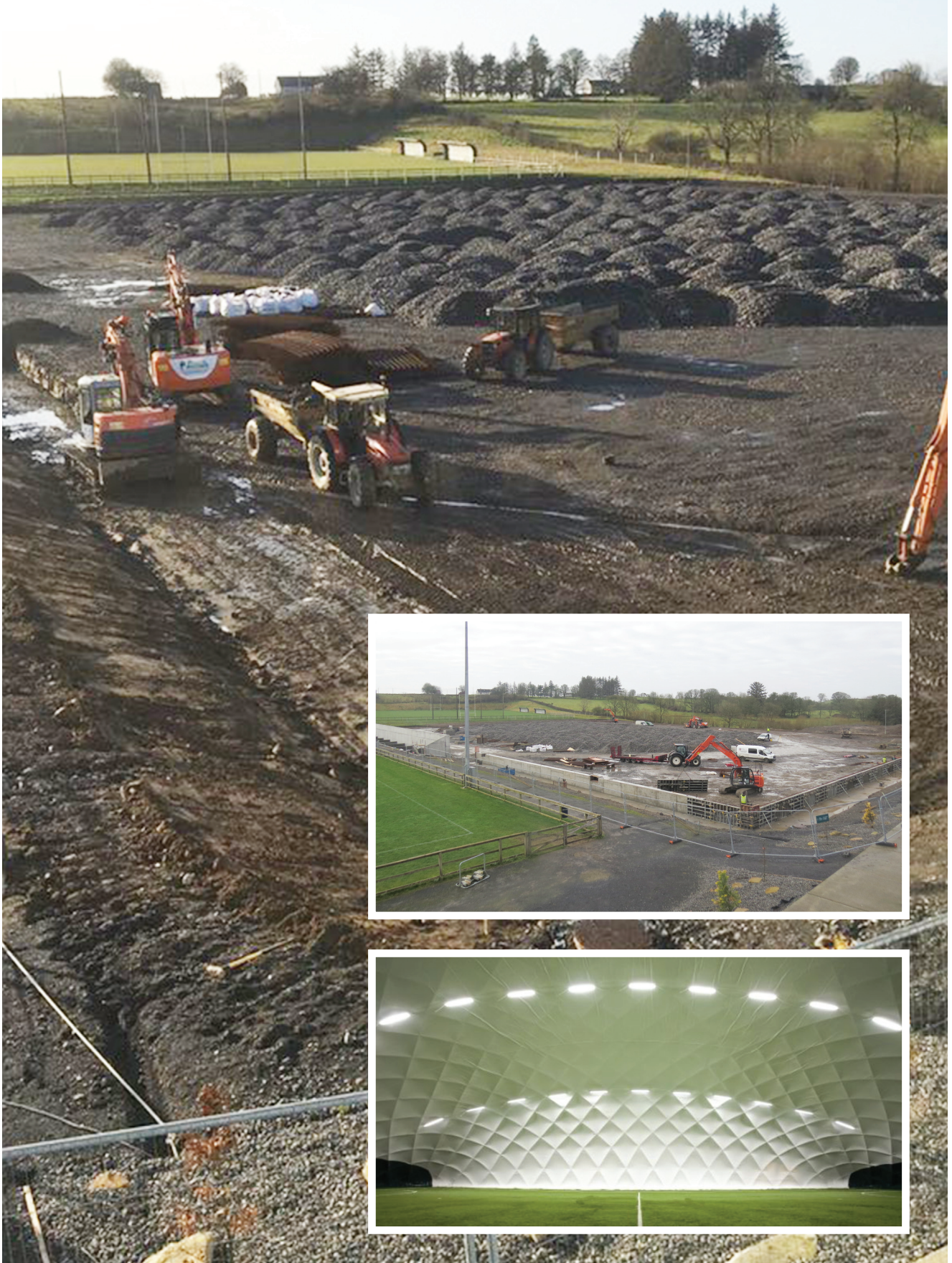
Ground work for the Air Dome.
